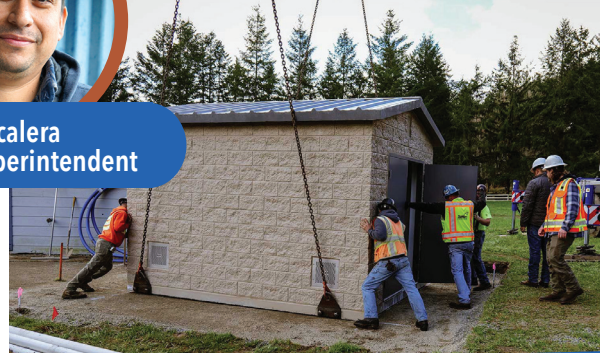
New Snow Creek wellhead building being placed.
