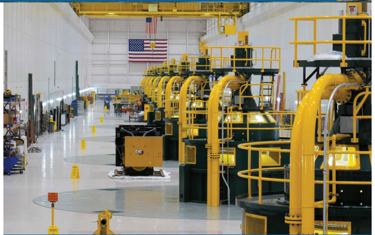
The Wanapum Dam powerhouse features 10 hydro generators.
