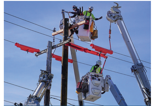
Line crew replace a 3-phase distribution pole in Port Townsend.
