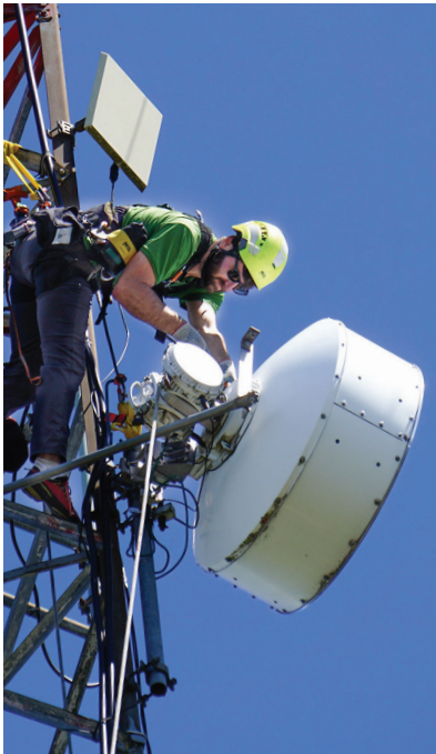
Climber removes old receiver from tower.
